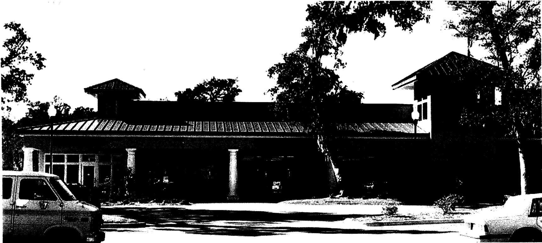
Example of covered walks with doric columns to disguise flat roof. Turrets are used to break up the long horizontals. Note the glass pattern
